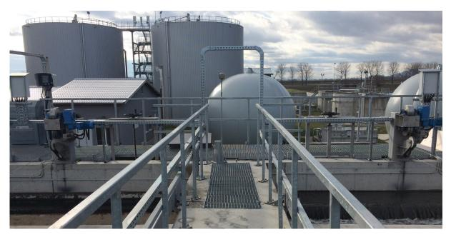
WWTP 2 Digester Biogas 21500 m³/d 2 x 1300 m³ Volume 1400 m³/day Cogen-Unit150 kW = 167 Wh/m³ WWBenchmark130 Wh/m³ electrical
